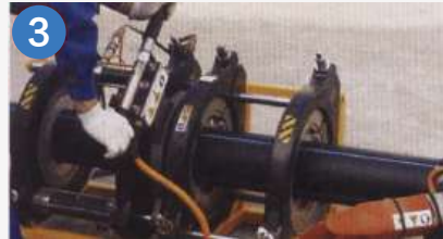
③ Put in the heating plate.
