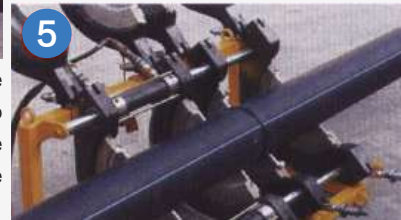
⑤ The hot melt is completed.
