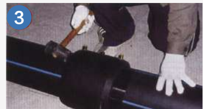
③ Place the electrofusion tube on the tube and straighten the tube to the same axis.
