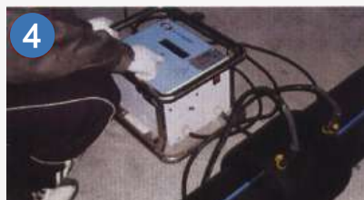
④ Conductive welding, there should be a little solution in the hole to be observed.
