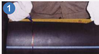
① Clean the dirt on the surface to be connected to the pipe and mark the insertion depth.
