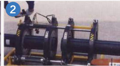
② Place the pipe to be connected on the welder fixture and clamp it, clean the pipe to be connected and mill the joint surface, and straighten the two butt joints so that the misalignment is no more than 10% of the wall thickness.
